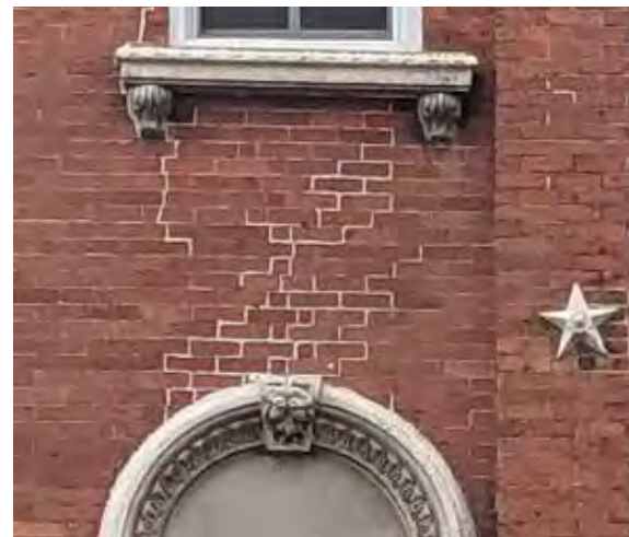
Incorrect use of mortar can impact the aesthetics and character of a building.
