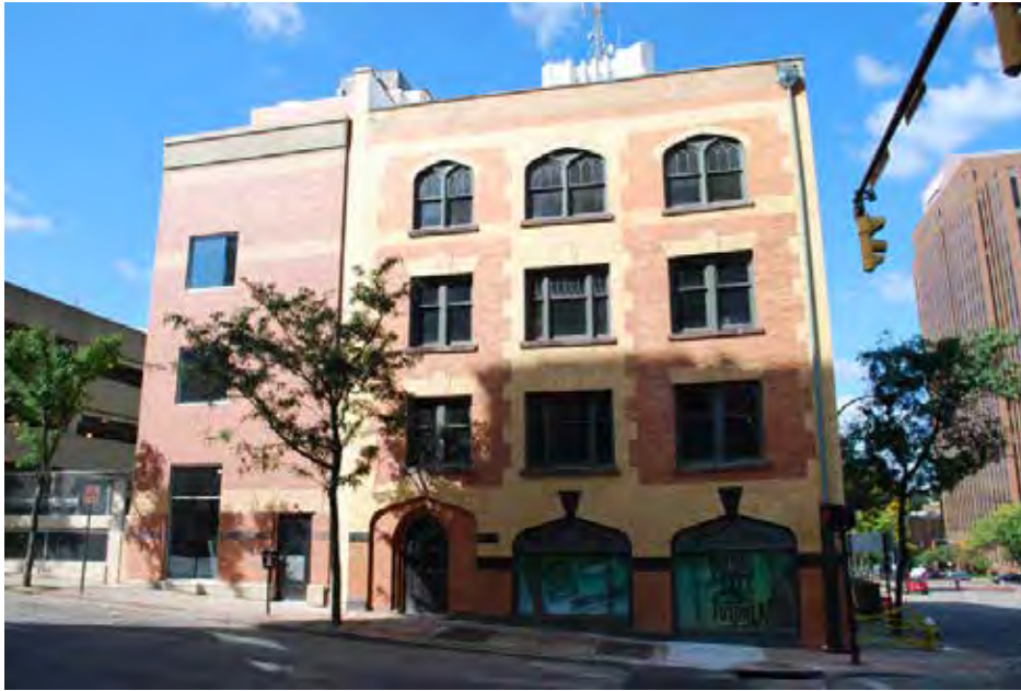
This photo shows the elements of continuity in brick bands of color and matching elevation of this urban infill's front façade (left). The addition houses a stair, therefore the windows align with the stair landings.
