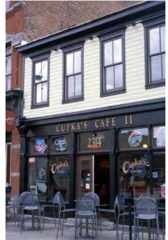
On buildings three stories or less, windows on primary (street facing) elevations should match in details and materials.
