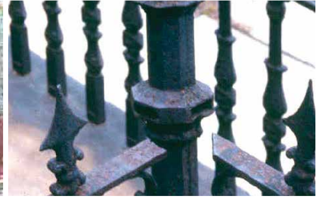
A corroded metal fence has failed at the connections between the railings and the post.
